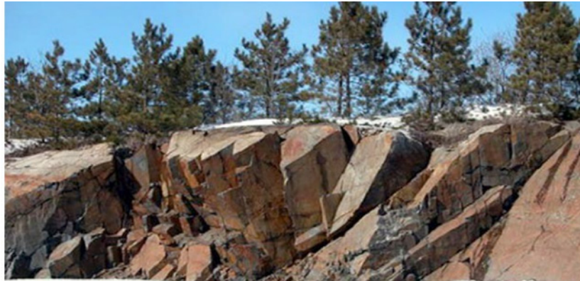
Figure 4: Note Hoek's own figure caption from Hoek and Diederichs, [15] which is an article about deformation modulus. 'Road cut in which the size of individual rock blocks is of the same order as the height of the cut. Rock mass classifications, based on the assumption of homogeneity, cannot be applied to this rock mass'. This Hoek advisory emphasises the gulf between GSI and the intended use of the Q-system which is obviously used to address just such rock masses, which are common, also in tunnelling. Refer to Figures 5 and 6 to see further problems.
